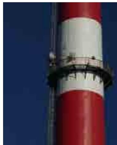
Fig. 7 Chimney after repair and reconstruction of warning coatings
