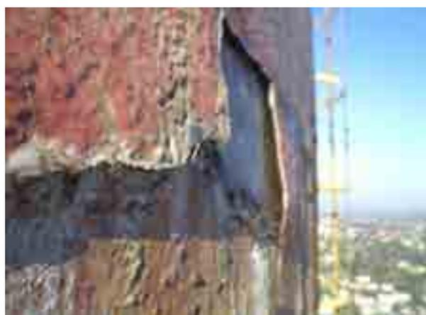
Fig. 5 Condensate degrading wall surface of the chimney [3]
