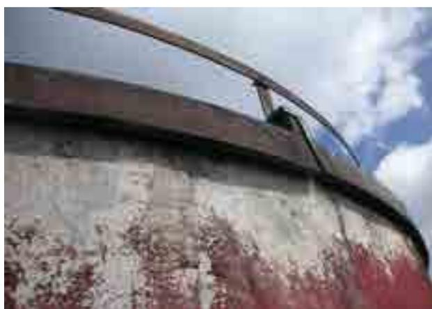
Fig. 4 Condensate degrading the chimney outlet
