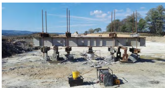
Fig. 1. Static Load Test (SLT) testing appliance anchored to adjacent piles
